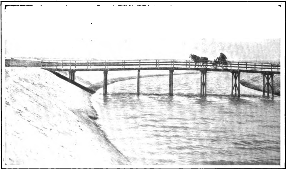
THE TWIN FALLS CANAL IS EIGHTY FEET WIDE AT THE BOTTOM OF THE DITCH. IT IS OVER SEVENTY MILES LONG AND IS THE LARGEST IRRIGATING CANAL IN THE WORLD
